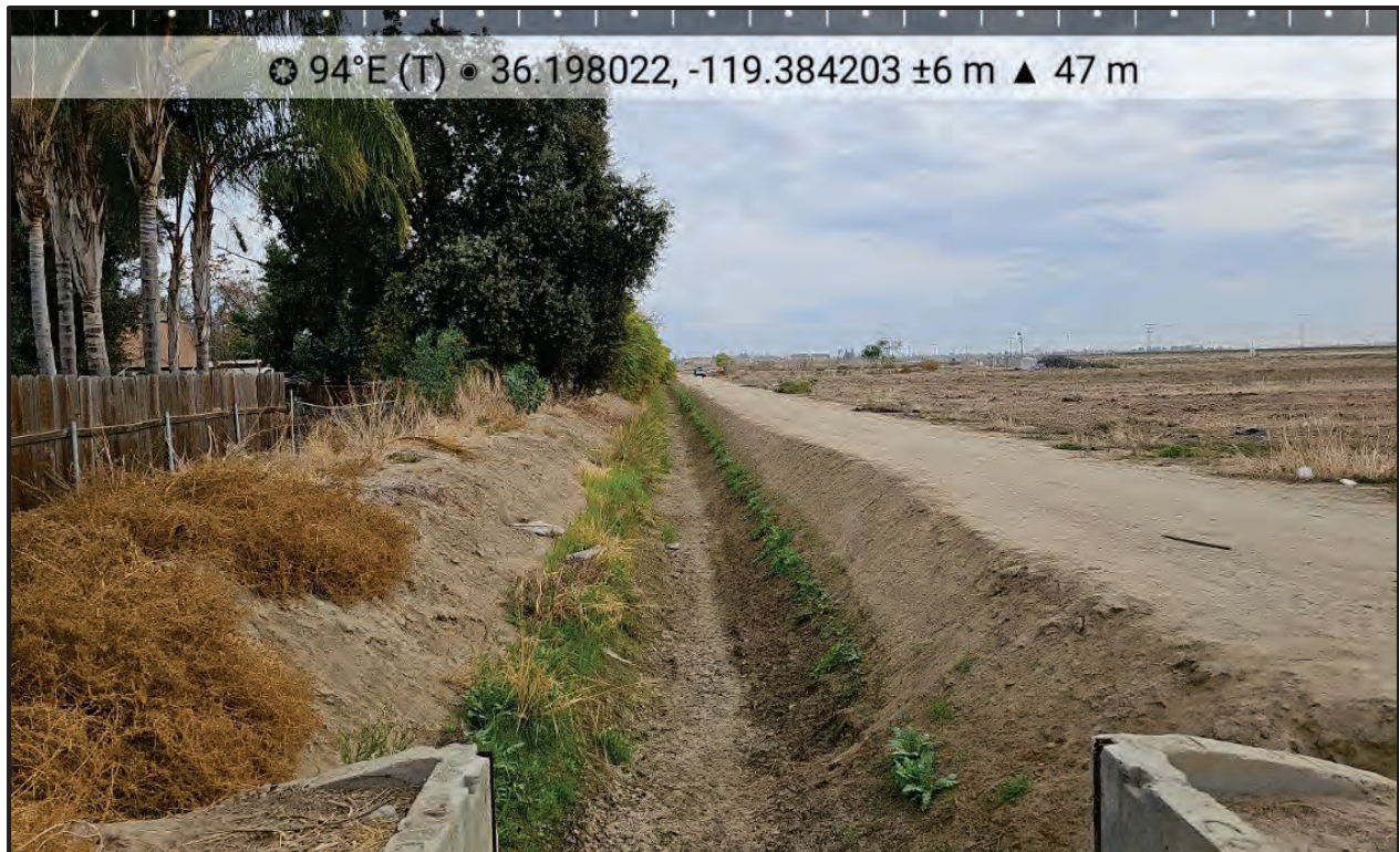
Photo 6: Drainage Ditch Along Northern Boundary
